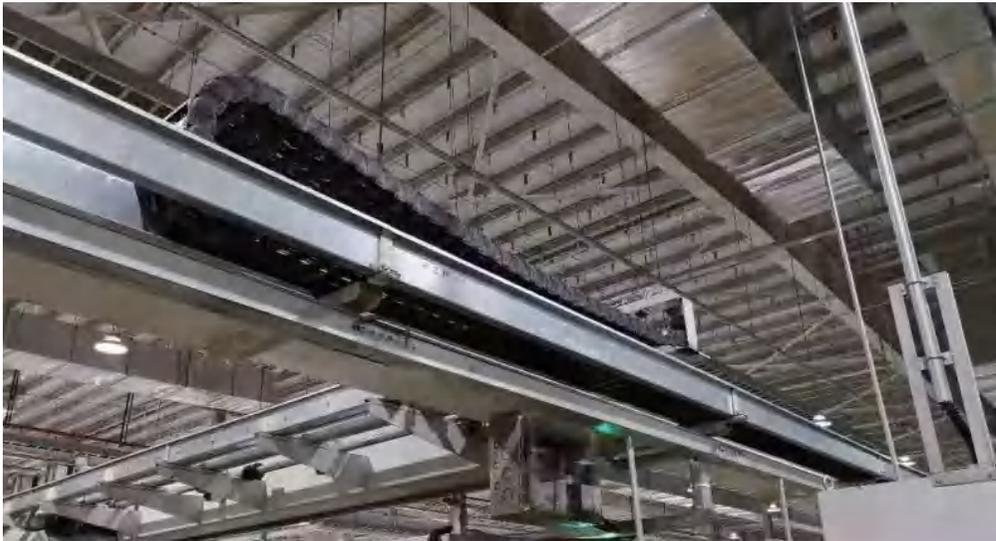
The Guide through system is an indispensable guiding device for the application of long-travel length energy chains.
